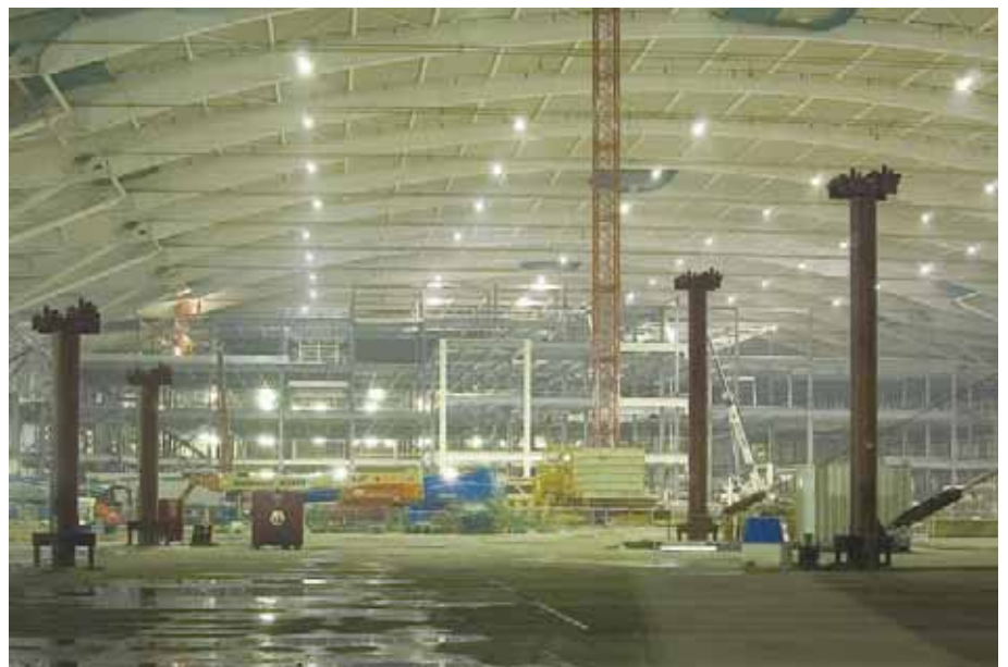
11. Central section clad and prestressed, May 2004.
