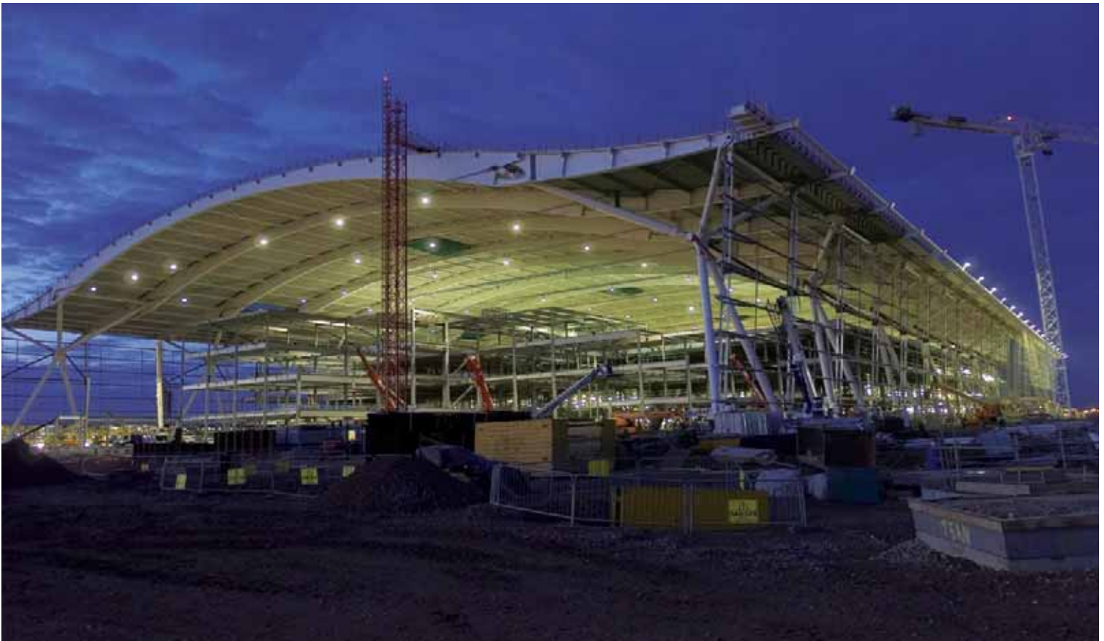
25. The main terminal building in summer 2005.
