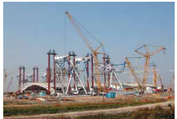
9. Roofing material in place prior to erection.
