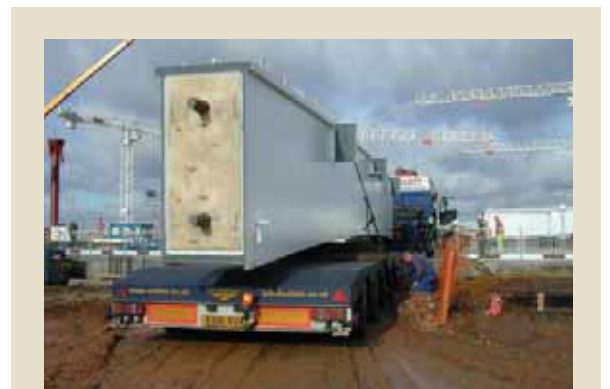
8. Rafter section arriving on site.
