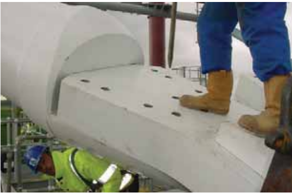
20. Connection of arm to torso.
