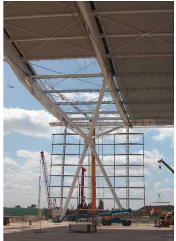
13. Bracing in roof plane and abutments.
