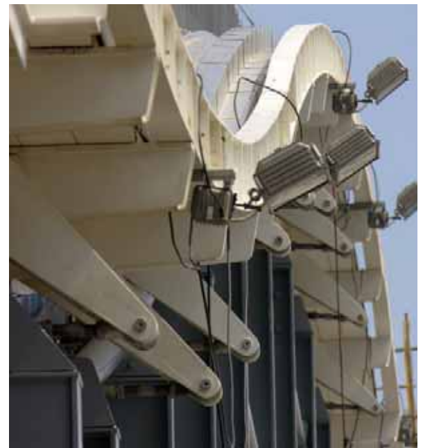
7. Joint at head of south façade.
