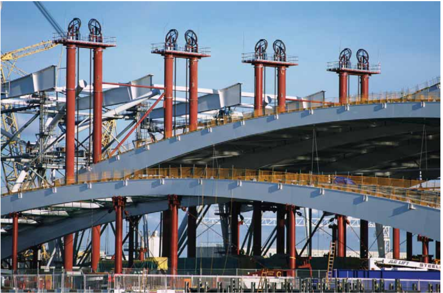
10. Jacking of roof elements.
